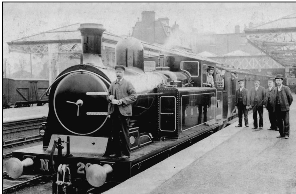
below: A spotless LD&ECR class A 0-6-2T no.26 stands at the head of a train at Chesterfield Market Place in Sept. 1906. It has been bulled up for Royal Train duty. The railway management on the platform are posed for a photograph along with the footplate crew. The driver with his oiling can takes pride of place. photo: John Alsop collection
